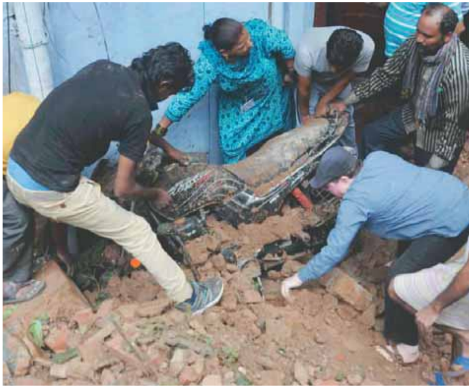
People busy in rescue work after house collapsed in Ganeshganj on Friday
